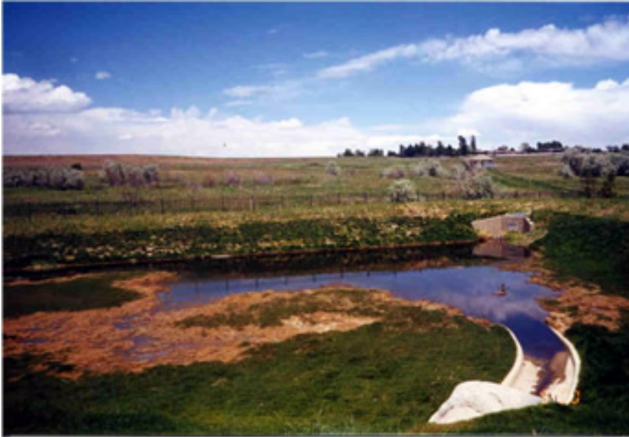
Grant Ranch EDB prior to construction of a micropool and energy dissipation.
