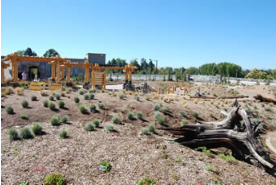
Mordecai Children's Garden Green Roof shortly following construction
