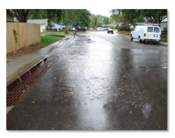
**Photograph 7-6.** Weir performance decay can be observed in this picture as flow appears to enter only the first two inlets while exceeding the height of the upstream curb.
