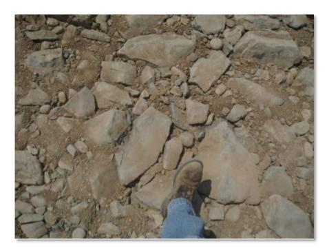
Photograph 8-21. Void-filled riprap after placement and compaction.
