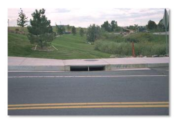
**Photograph 7-5.** Inlets that are located in street vertical sag curves (sumps) are highly efficient.
