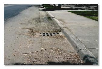
**Photograph 7-6.** Clogging is an important consideration when designing inlets.
