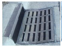
(a) CDOT Type 13 grated inlet in combination configuration
