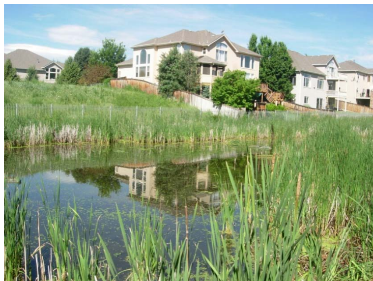
Photograph CWP-1. This constructed wetland pond, located downstream of an extended detention basin, is part of a BMP "treatment train."
