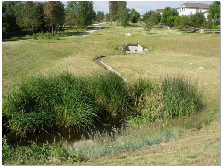
Photograph EDB-1: This EDB includes a concrete trickle channel and a micropool with a concrete bottom and grouted boulder sideslopes. The vegetation growing in the sediment of the micropool adds to the natural look of this facility and ties into the surrounding landscape.
