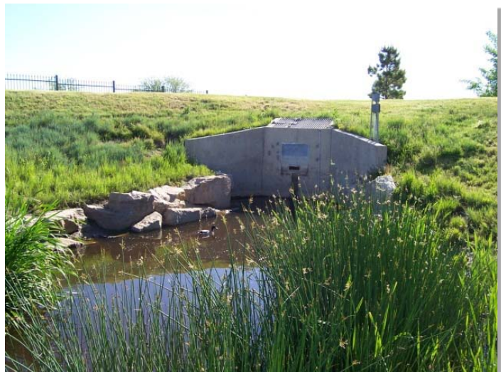
Photograph EDB-2. The initial surcharge volume of this EDB is contained within the boulders that surround the micropool.
