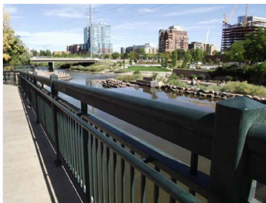
Photograph 10-8. At Confluence Park a rub rail was included as part of the rail design. This, in addition to the 14-foot path width, improves safety in this high-use area.
