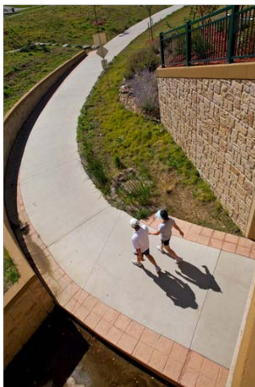
Photograph 10-4: Rumble strips warn the user of the path edge without reducing capacity for flood flows. Photo Courtesy Architerra Group.
