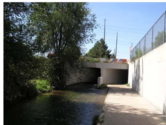
Photograph 10-16. Multi-cell culverts can be uninviting, especially if the user is not able to see the other end.
