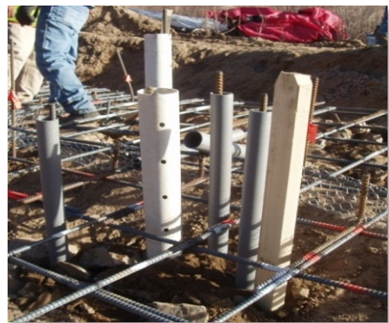
Photograph 9-17. Small vegetation pockets can be formed using PVC, lumber, or other items. Removed these items shortly before or after the concrete cures. If done after the concrete cures, coat the items with a lubricant to facilitate removal.
