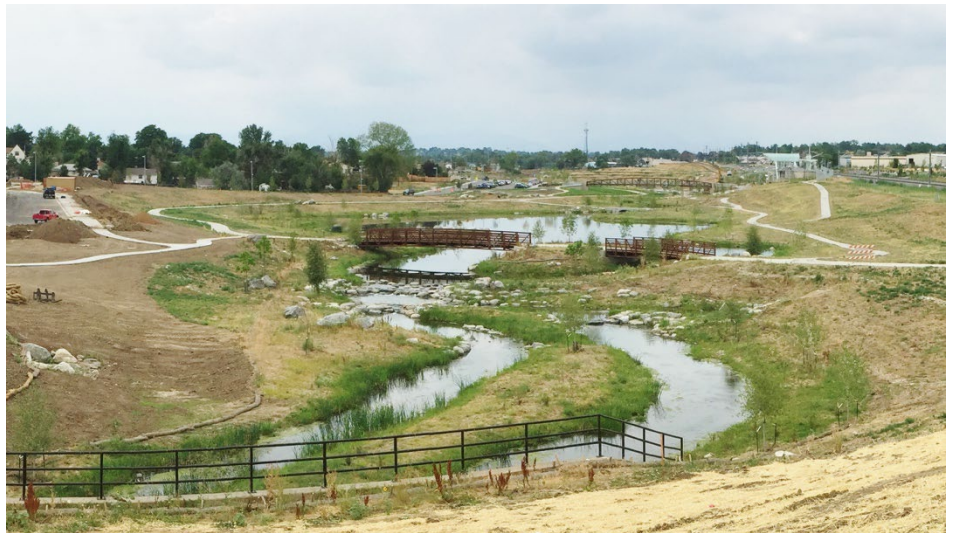
Photograph 11-7. Bridges for a shared-use path.
