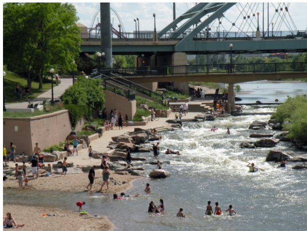
Photograph 10-38. Multi-use design of the whitewater bypass at Confluence Park conveys flood flows, offers continual access, and avoids overly-retentive hydraulic jumps over a wide range of flows. Photo courtesy of Thanis McLaughlin.
