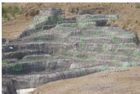
Photograph 9-26. Spray paint is used on the “skim coat” of a sculpted concrete structure prior to concrete placement to identify the locations for fracture lines and other features.
