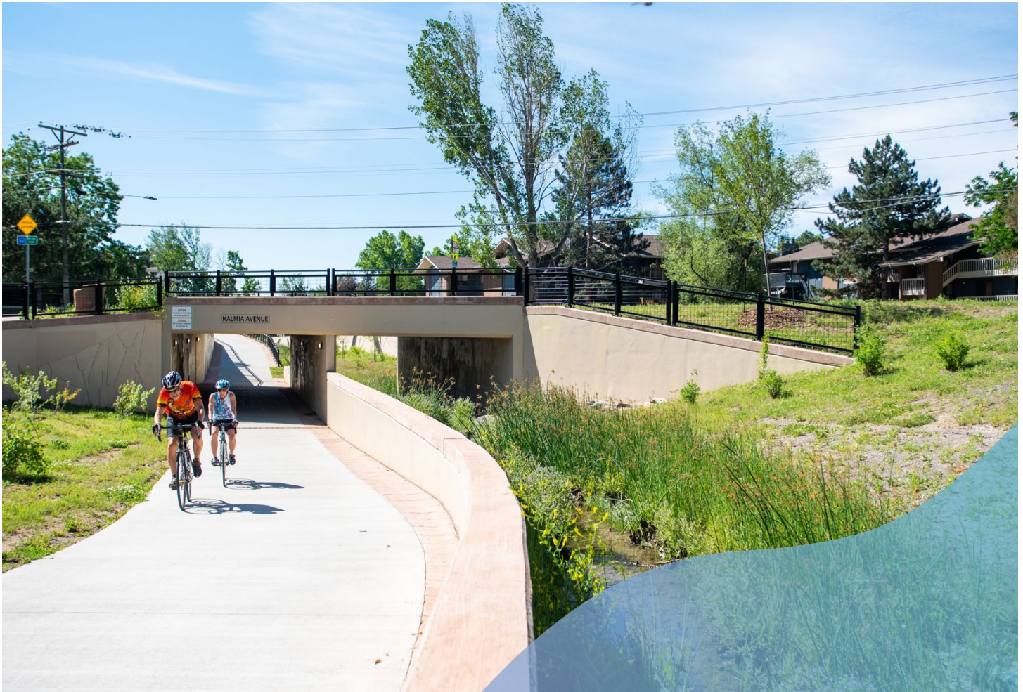
Photograph 11-1. Single-cell box culvert structure with recreational path set above minor flood elevation
