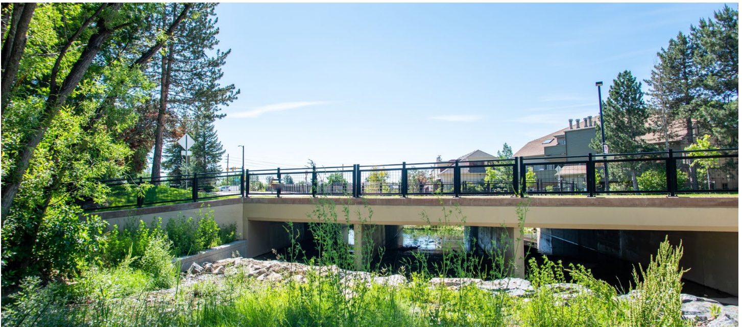
Photograph 11-3. A three-cell box culvert on Wonderland Creek.
