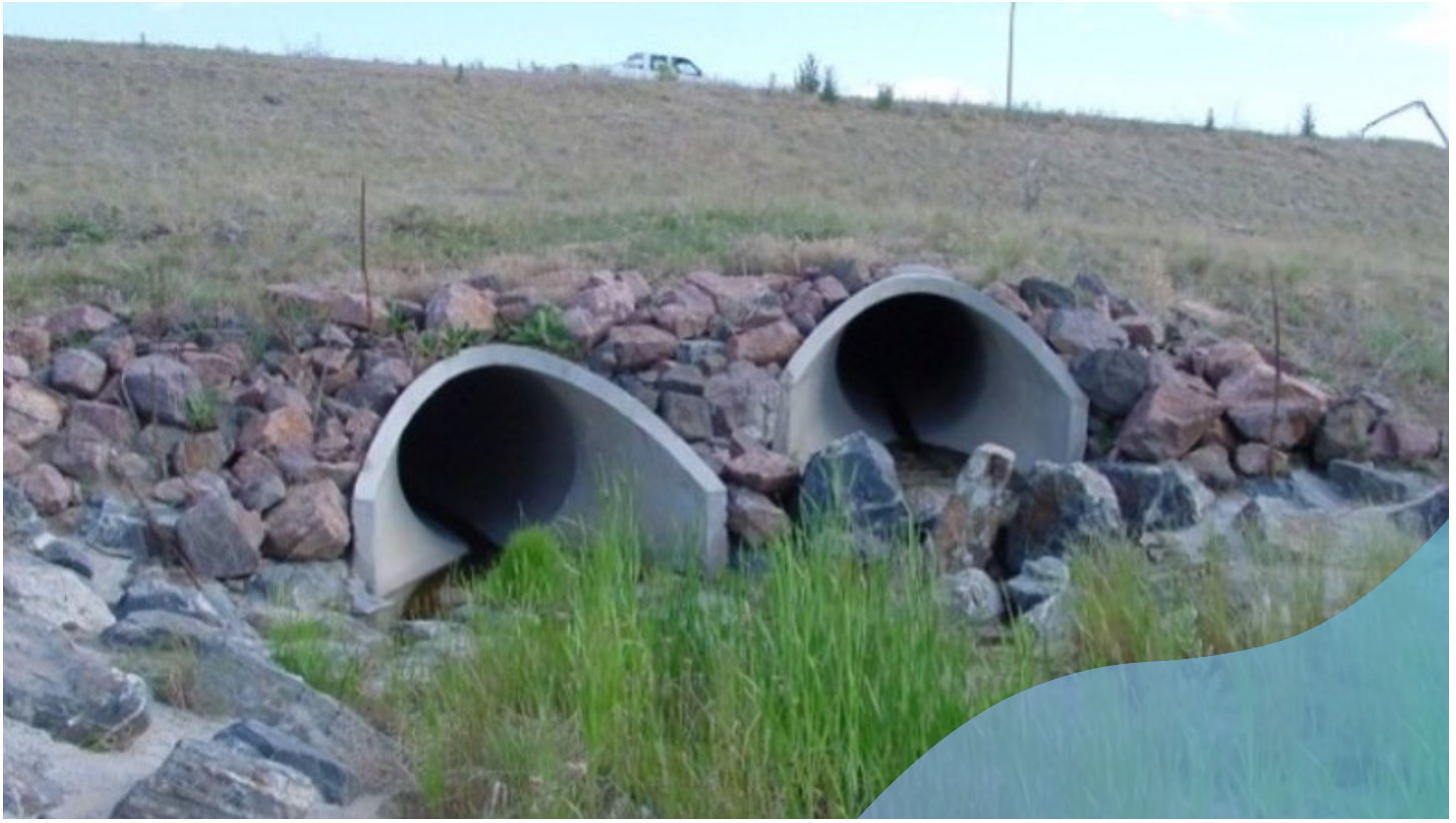
Photograph 11-6. Energy dissipation and outlet protection are essential to promote channel stability.
