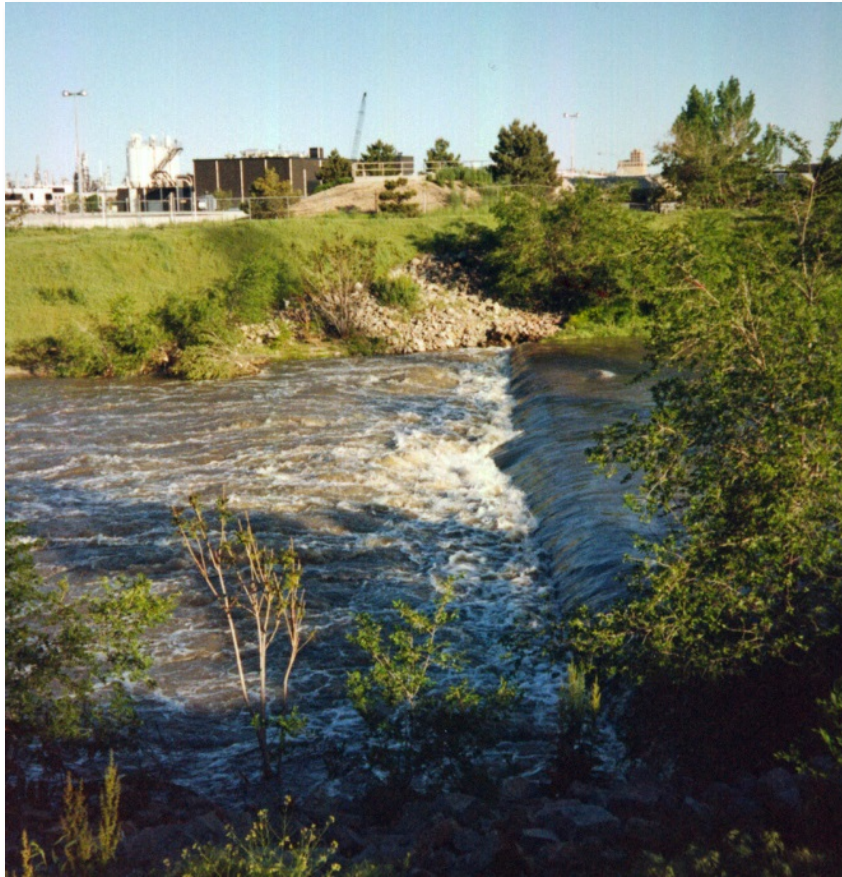
Photograph 10-34. Currents downstream of dams or even drop structures can create an overly-retentive hydraulic jump that can trap in-channel users. Sometimes called “keepers” or “drowning machines,” these hydraulic conditions can be deceptively dangerous. The misleadingly dangerous structure shown here created this condition with only 1.5 feet of hydraulic drop before UDFCD retrofitted it to be safely boatable.
