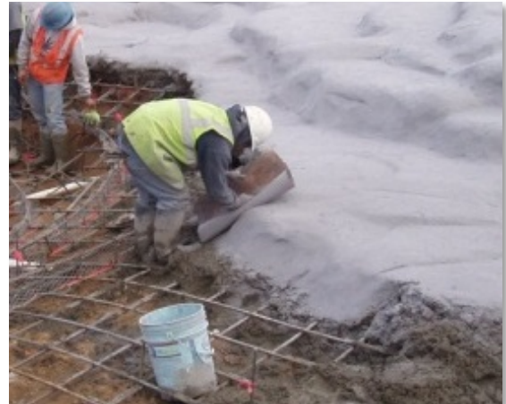
Photograph 9-15. Texturing a sculpted concrete drop with a rubber skin.
