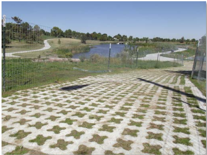
Photograph 10-26. Reinforced grass pavement shortly after construction.
