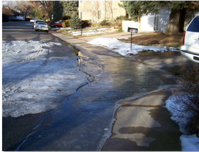
Photograph 7-7. The location of inlets is important to address the effects of nuisance flows.
