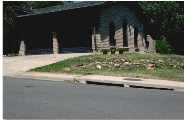
Photograph 7-4. Gutter/street slope is a major design factor for both street and inlet capacity.
