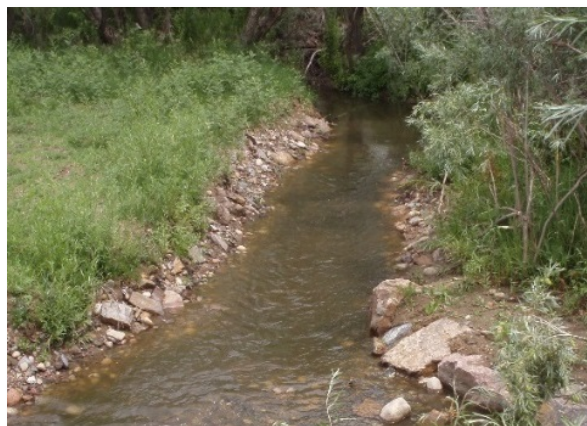
Photograph 8-17. Void-filled riprap used to stabilize the low-flow channel.
