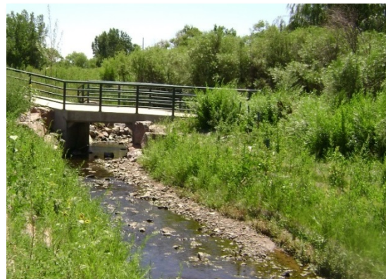
Photograph 8-16. (Same view as photo 8-15 taken one year following construction.)
