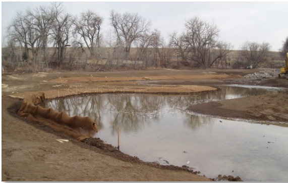
Photograph 8-13. Coir blanket used to protect the outside banks of a low-flow channel immediately following construction.
