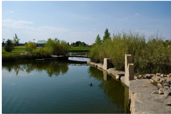
Photograph 1-5. Retention ponds with permanent ponding have many benefits, including flood reduction, water quality and land values.
