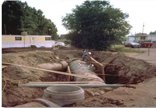
Photograph 7-2. The capital costs of storm drain construction are high, emphasizing the importance of sound design.
