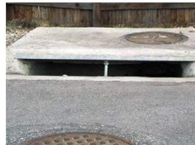
(c) CDOT Type R curb-opening inlet
