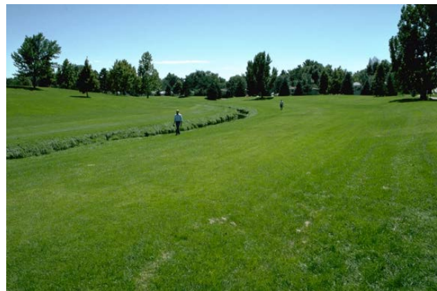
Photograph 3-6. A wide, open waterway carries floodwater at modest depths while maintaining low velocities to inhibit erosion.
