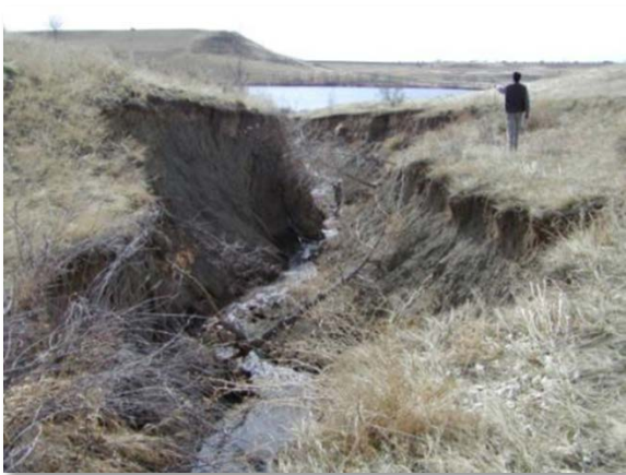
Photograph 8-7. Degraded channel (before restoration).
