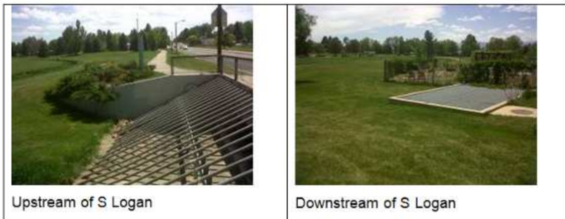
Figure 3-3 Crossing Box Culvert under S. Logan Street
