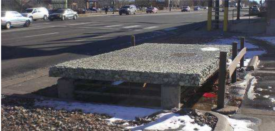
Figure 4-2 Entrance Inlet at Colorado Blvd and Yale Street
