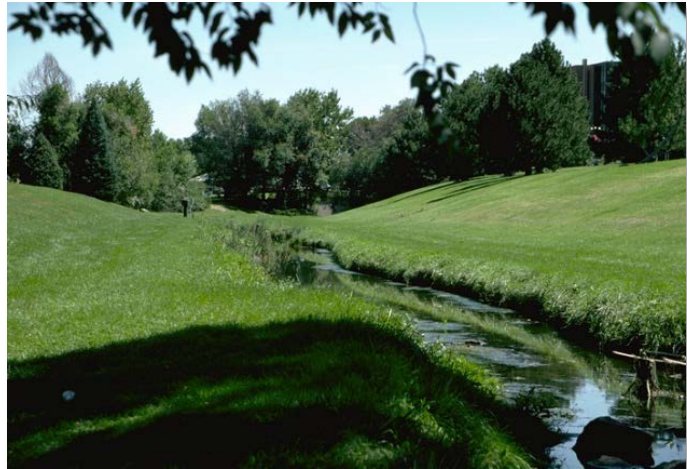
Photograph 1-1. Local grass channel after 35 years of service. Ann Spirm of the Massachusetts Institute of Technology refers to this channel as “urban poetry” in her publications.
