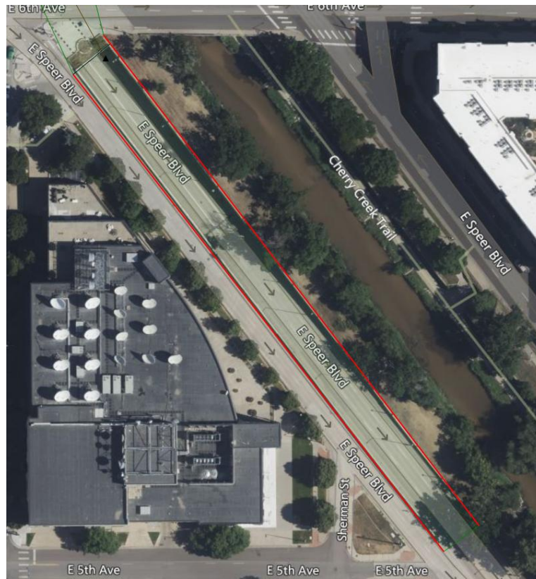
Figure 19 Example of a Wall along a Roadway Tunnel Approach
