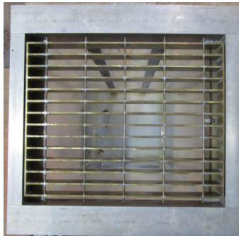
Figure 8 - Plan view of CDOT close-mesh grate
